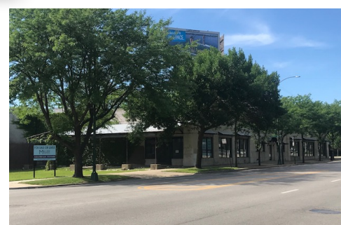
6834-6868 N Western Avenue, Chicago, IL 60645
