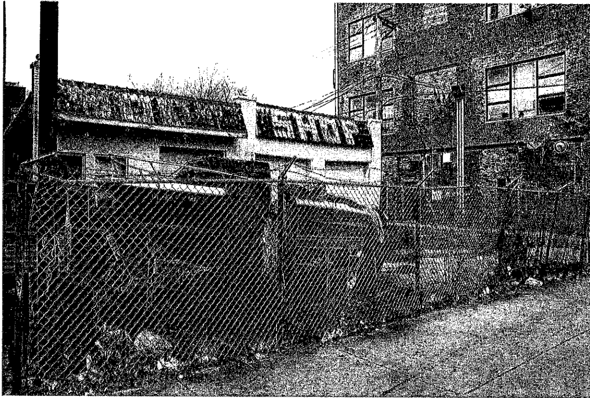
Subject Property as view from the Southeast
