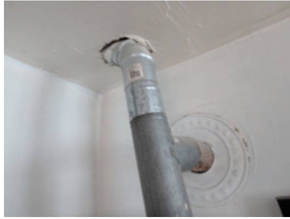
Typical older space heater with less than ideal flue pipe set up, typical deterioration at unit
