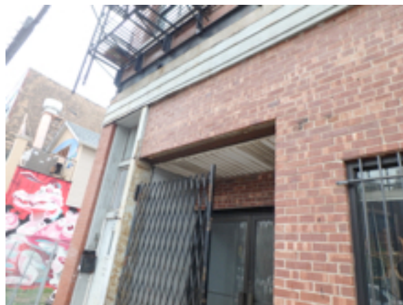
No signs of sagging at doorway lintel
