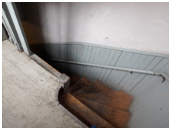
Missing guardrail at stairway
