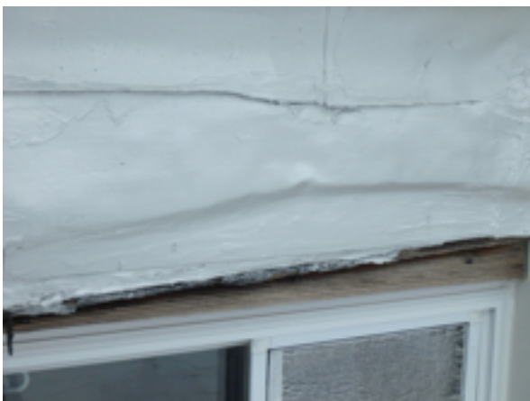
Less than ideal roof to window terminations, will likely lead to rot out at tops of windows
