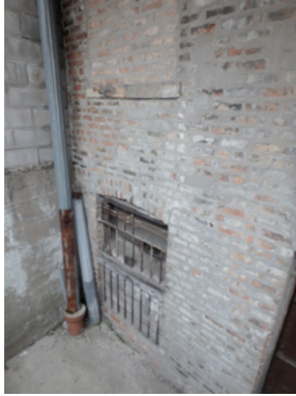
Rusted out downspout likely flooding pad area
