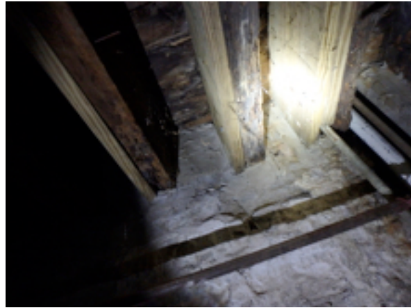
Termite type damage at multiple wood joists and poor sistering work
