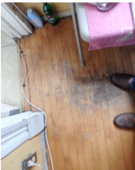
Some floors look ok, some floors a bit rough, sanding and refinishing should be fine
