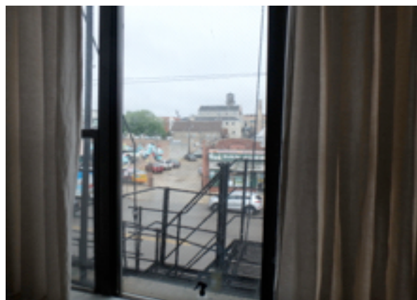
If the fire escape remains in place, wired glass window assemblies need to remain in place as well
