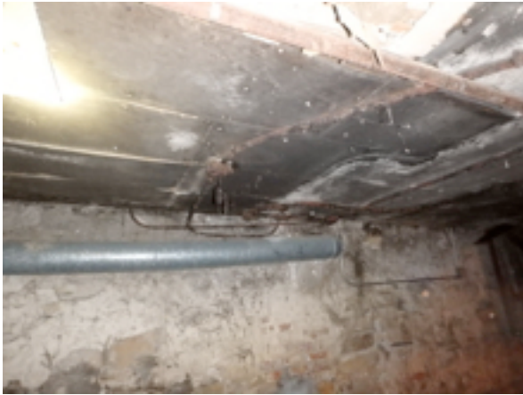
Typical poor ceiling conditions, all needs to be stripped up to joists
