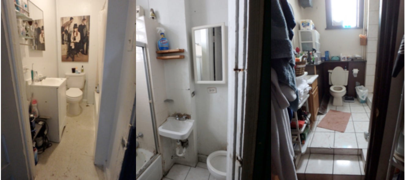
Typical bathroom views
