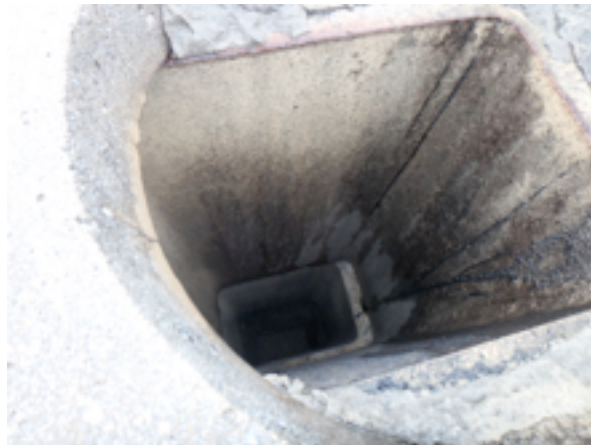
Typical shifted clay liner sections
