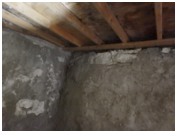
Heavy water saturation, rot and wall deterioration signs under grade level pad
