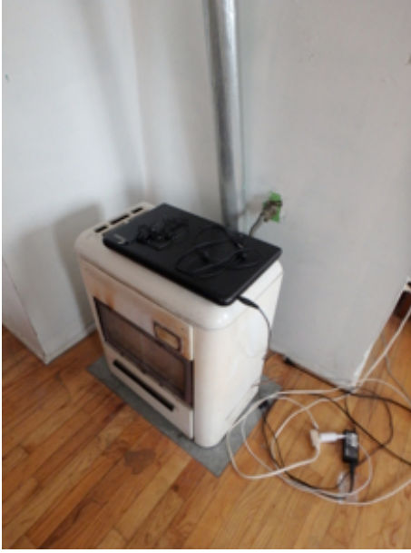
Typical older space heater with less than ideal flue pipe set up, typical deterioration at unit
