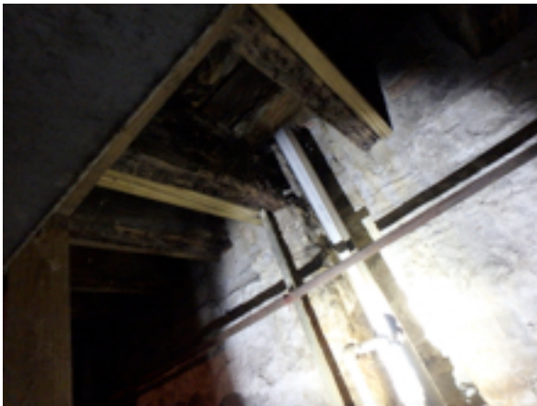
Joists and mid span supports will all need extensive carpentry repairs
