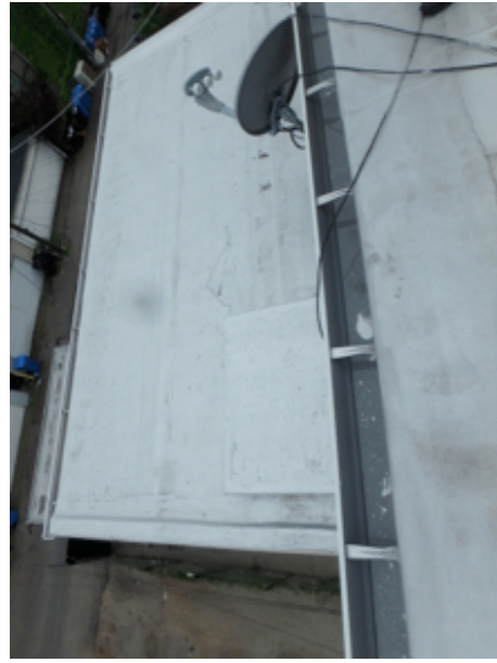
Rear porch roof view, overall ok
