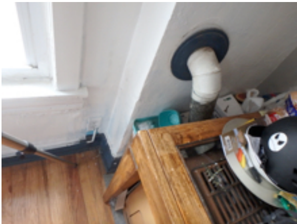
4 th floor apartment space heater in Dangerous & Hazardous condition, flue pipe disconnected at back of unit and open to wall; DO NOT allow tenant to use
