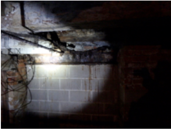
Front CMU wall with extensive rust and water intrusion signs
