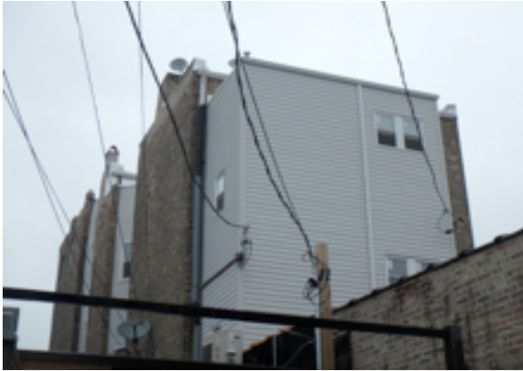
Rear of building view with enclosure
