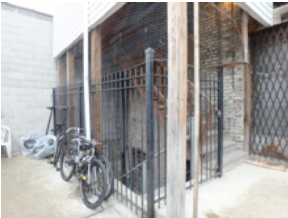
Rear of building entry area
