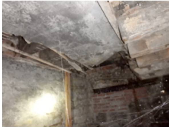
Typical poor ceiling conditions, all needs to be stripped up to joists
