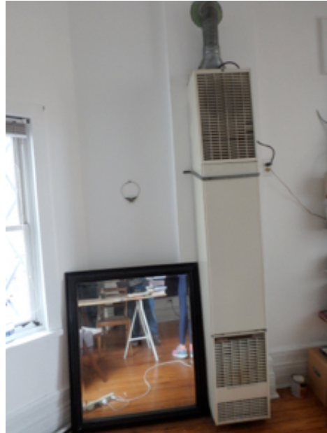
Space heaters dirty, poor flue pipe configurations, unit positions don't provide for good distribution
