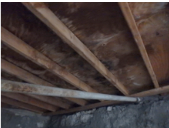
Heavy water saturation, rot and wall deterioration signs under grade level pad
