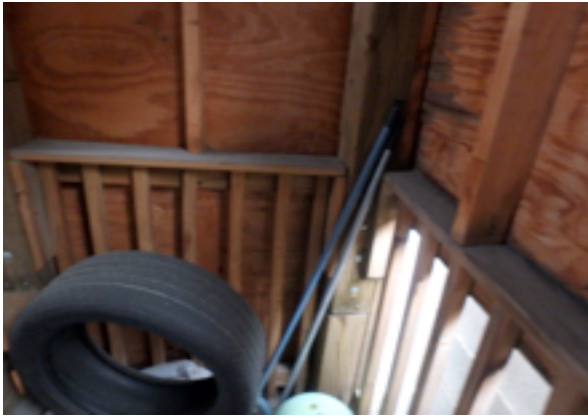
Lots of water intrusion and rotted plywood signs at rear porch enclosure
