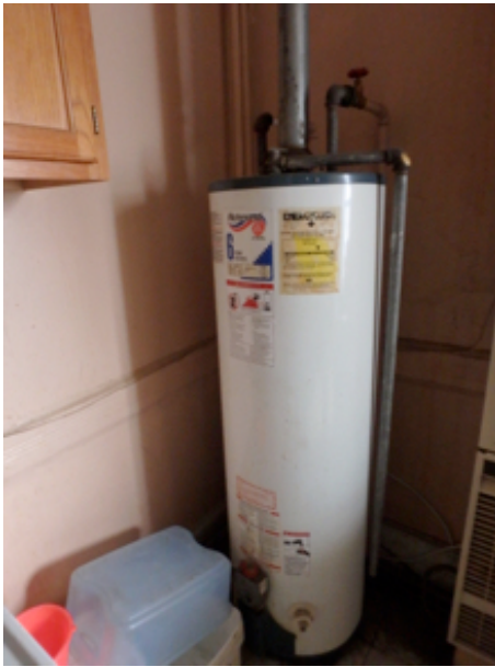
Typical water heaters in kitchens and closets, budget for full replacements
