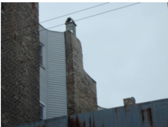
W elevation view, wall mostly ok but parapets need work
