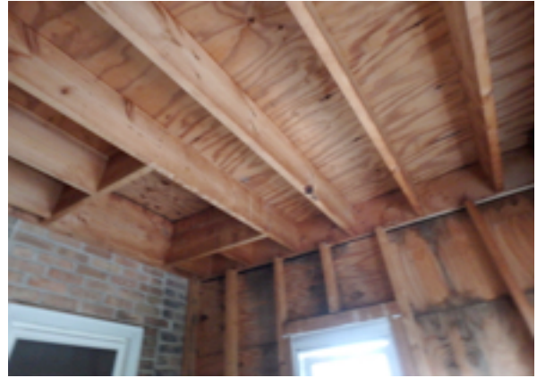
Lots of water intrusion and rotted plywood signs at rear porch enclosure
