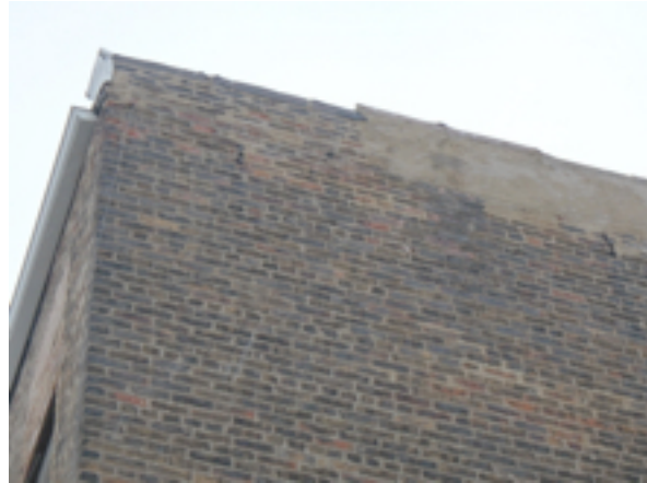
E elevation view, masonry mostly ok, parapet wall needs servicing
