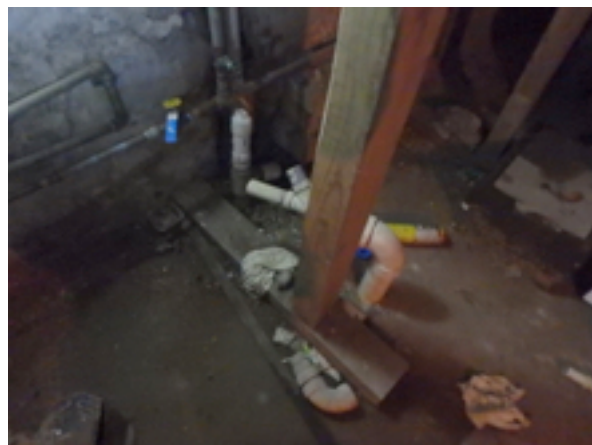
Basement bathroom and plumbing with non-compliant PVC piping
