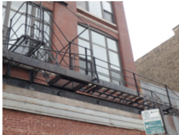
Fire escape views, fire escape was not accessed during inspection, no signs of pull out
