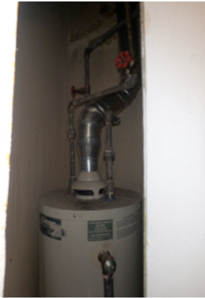
Typical water heaters in kitchens and closets, budget for full replacements
