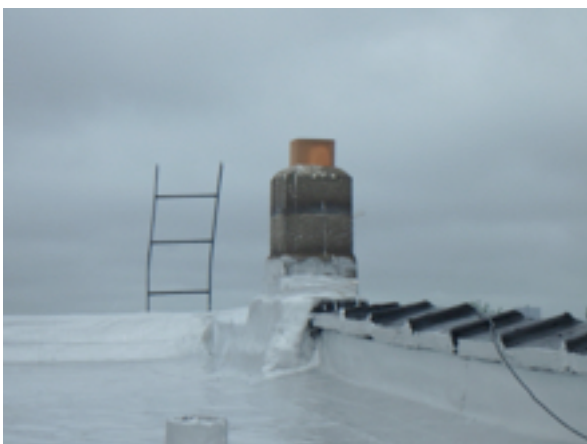
Chimney views, these block chimneys need rain hats and proper caps to keep water out of the long term
