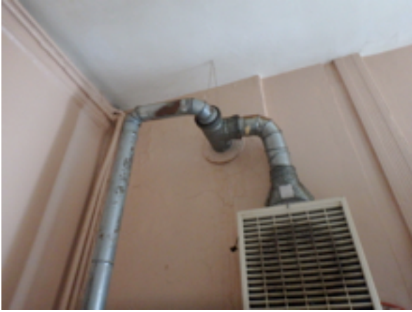
Space heaters dirty, poor flue pipe configurations, unit positions don't provide for good distribution
