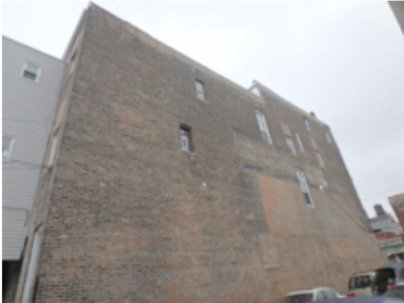
E elevation view, masonry mostly ok, parapet wall needs servicing
