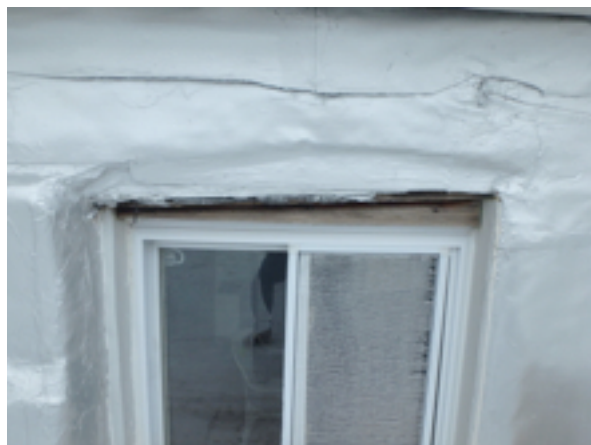
Less than ideal roof to window terminations, will likely lead to rot out at tops of windows
