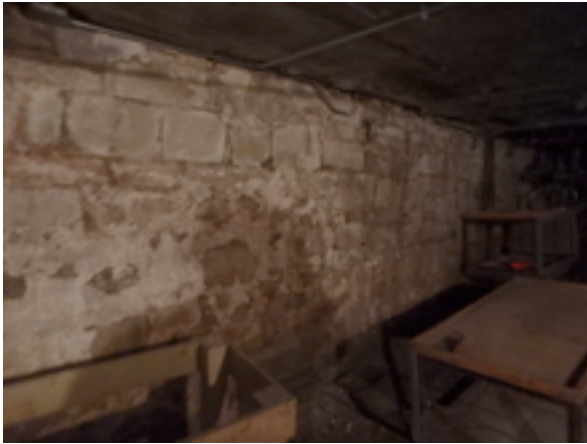
Typical old stone foundation walls with erosion
