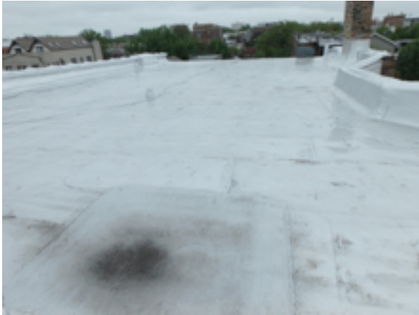
General roof views, some wrinkled and bubbles not no major heaving
