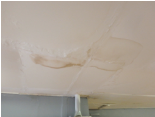
Typical water damage likely from plumbing leaks
