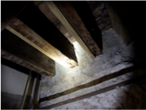
Termite type damage at multiple wood joists and poor sistering work
