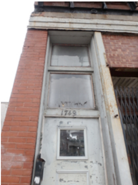
No signs of major movement at doorway, typical repairs should be fine
