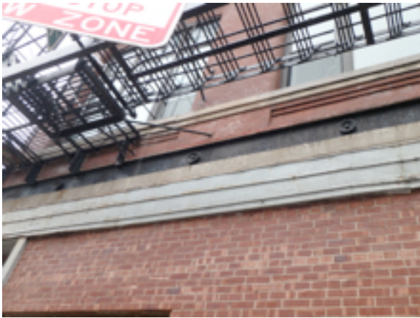
Main beam views and poor wall cover conditions at face wall
