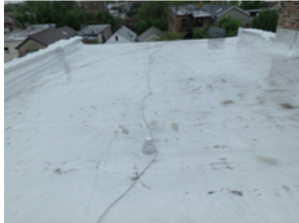
General roof views, some wrinkled and bubbles not no major heaving
