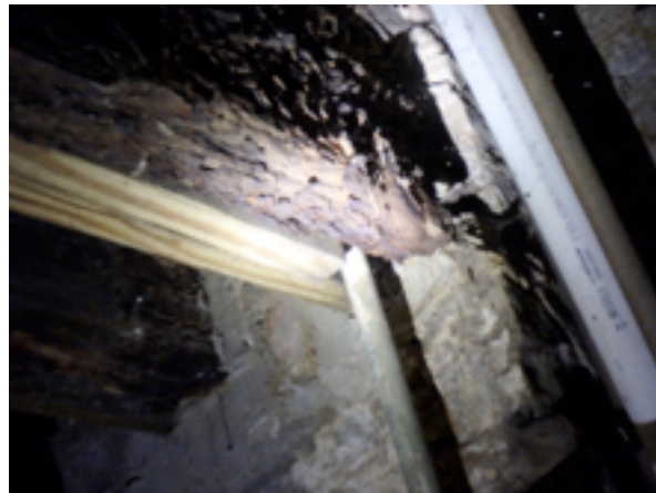
Joists and mid span supports will all need extensive carpentry repairs
