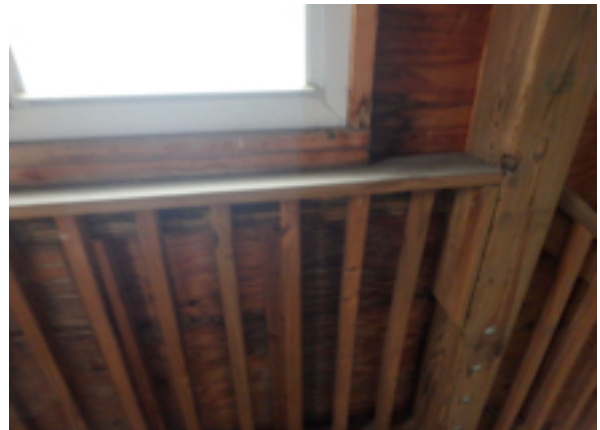
Lots of water intrusion and rotted plywood signs at rear porch enclosure
