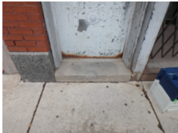
No signs of major movement at doorway, typical repairs should be fine
