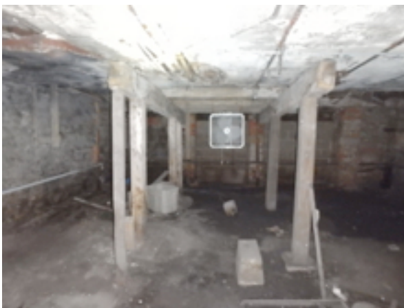
View towards front of basement
