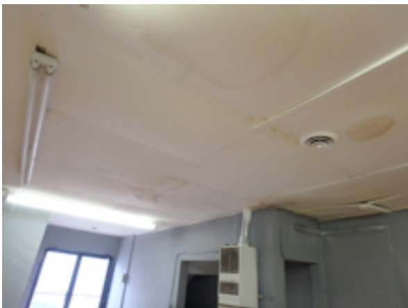
Storefront ceiling with water damage
