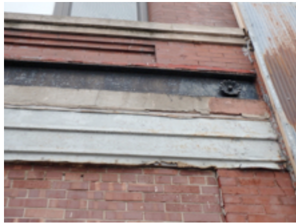
Main beam views and poor wall cover conditions at face wall
