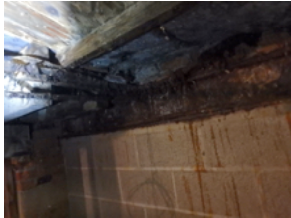
Front CMU wall with extensive rust and water intrusion signs
