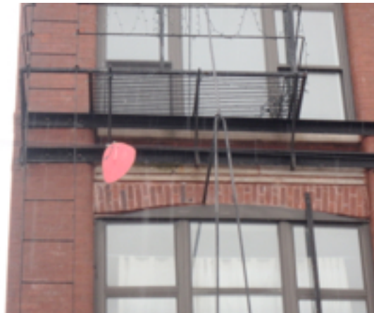
Fire escape views, fire escape was not accessed during inspection, no signs of pull out
