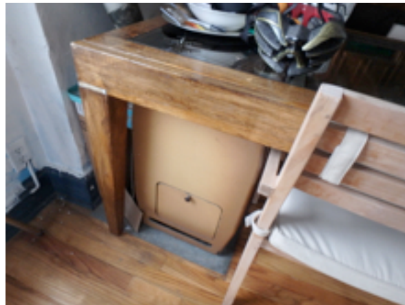
4 th floor apartment space heater in Dangerous & Hazardous condition, flue pipe disconnected at back of unit and open to wall; DO NOT allow tenant to use
