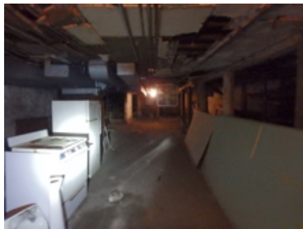
Rear basement area
