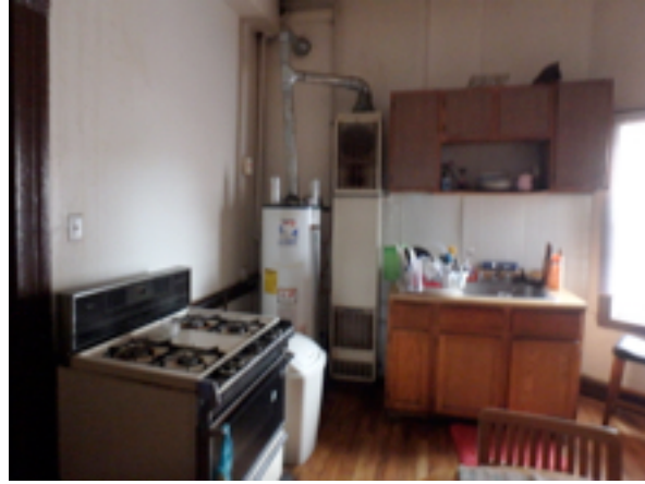
Space heaters dirty, poor flue pipe configurations, unit positions don't provide for good distribution
