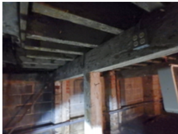
Rotted mid span beam, various additional support added at front of basement
