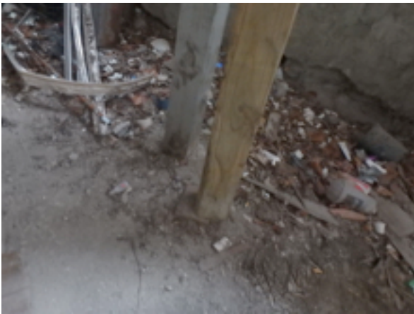
No post bases and very dirty conditions
