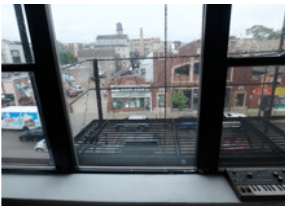
If the fire escape remains in place, wired glass window assemblies need to remain in place as well
