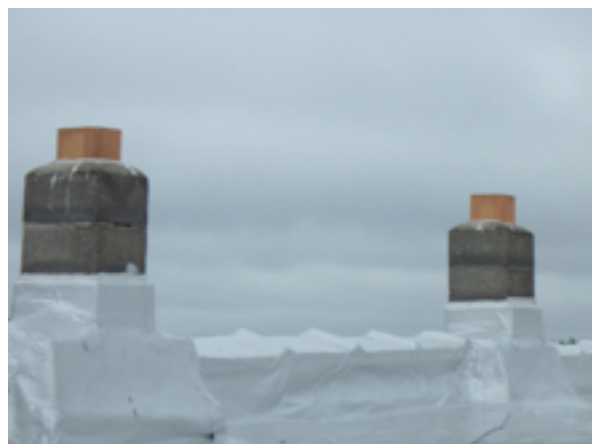
Chimney views, these block chimneys need rain hats and proper caps to keep water out of the long term
