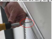
Once the screws are removed, you can remove the grille by pulling the top towards you
