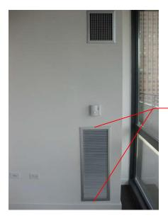
Fan Coil Return Air Grille. One screw on top and one on the bottom of grille.
