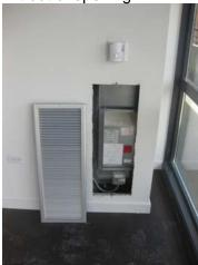
Remove the existing filter. Keep in mind it will have dust and dirt trapped in it so it may be messy. It may be a good idea to do this over a tarp or if you remove it while it is inside a garbage bag so the dust does not go all over your condo.
